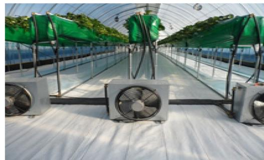
(b) Fan coil unit and double layer plastic duct
