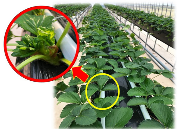
Fig. 2. The picture of crown heating piping installation.
