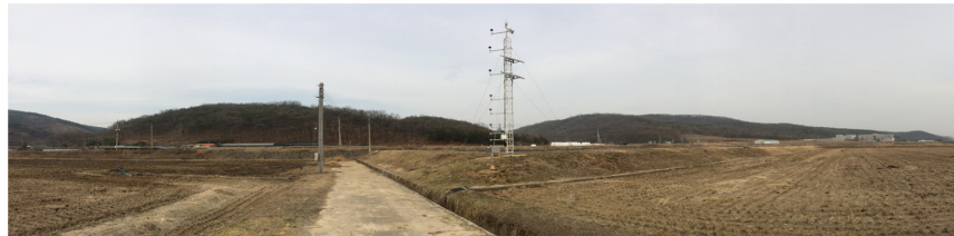
(a) Photographic views around the tower
