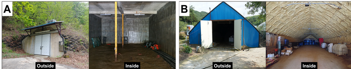
Fig. 1. Types of semi-underground warehouses including cave shape (A) and slanted shape (B) located on Gangwon Province in Korea.
